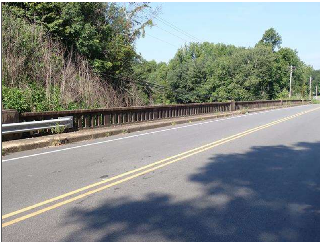
left bridge rail
