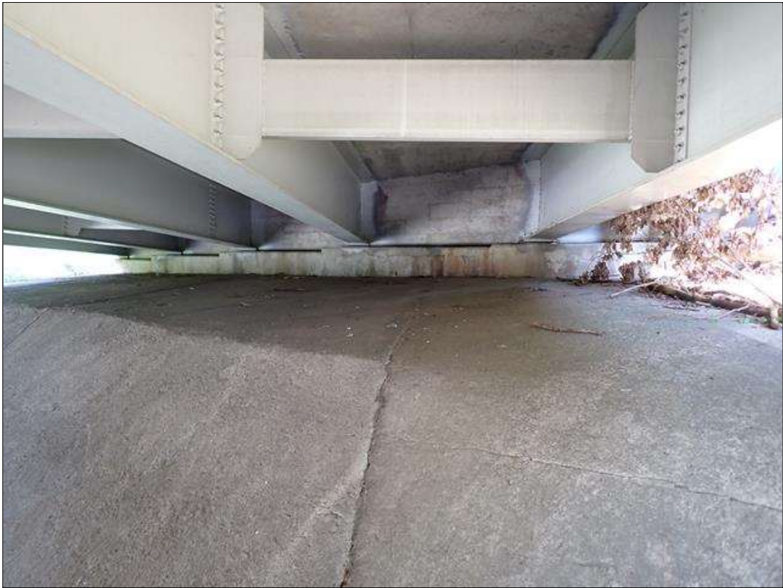
end bent 2 and slope protection
