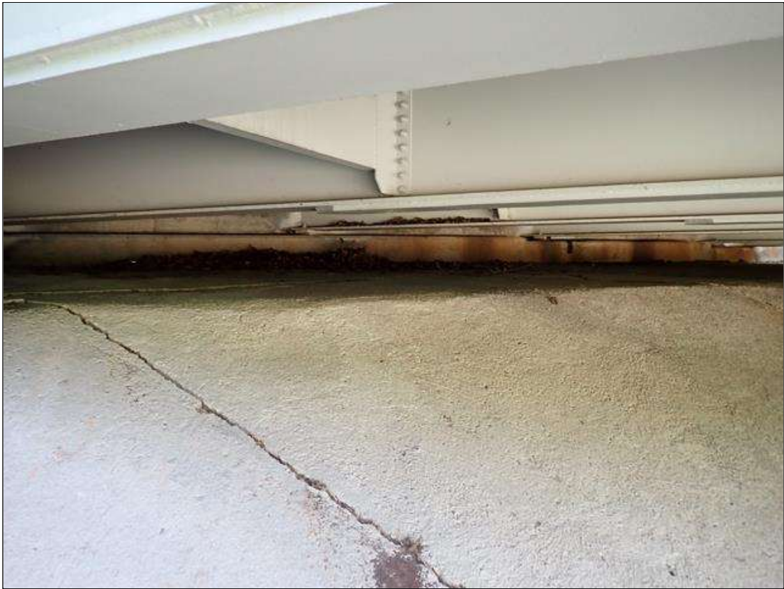
end bent 1 and slope protection
