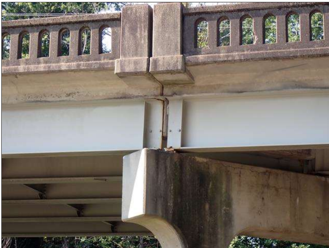
beams over bent
