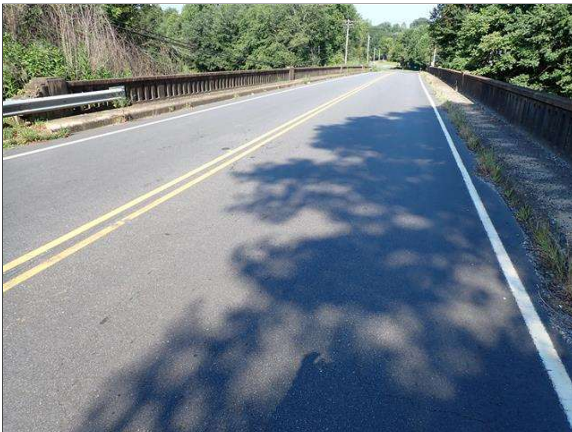
asphalt wearing surface
