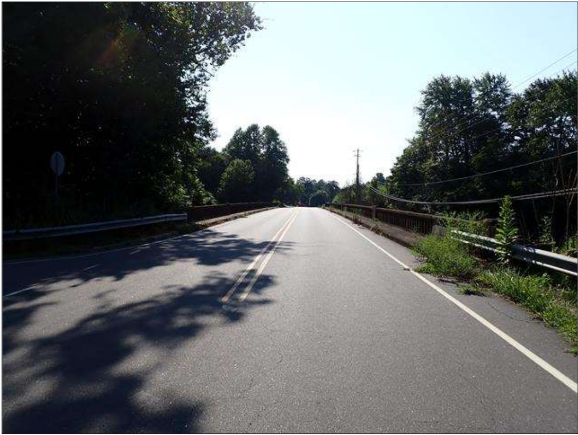
north approach looking south
