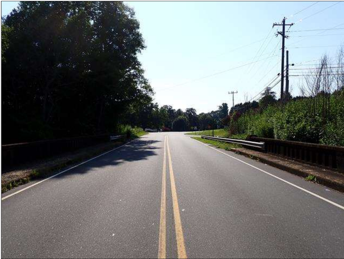
south approach looking south
