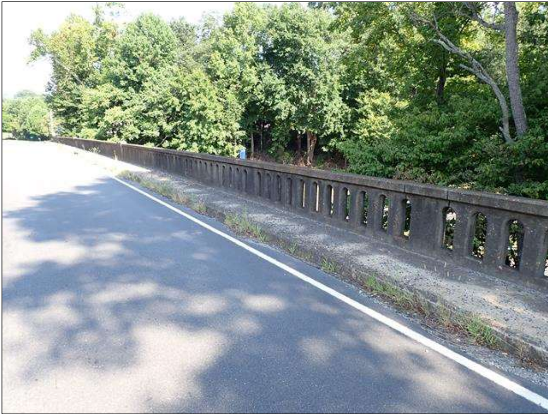
right bridge rail
