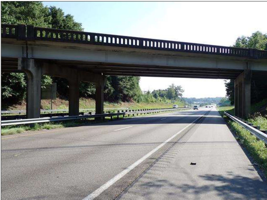
roadway under span 2, looking east (I-40 eastbound)
