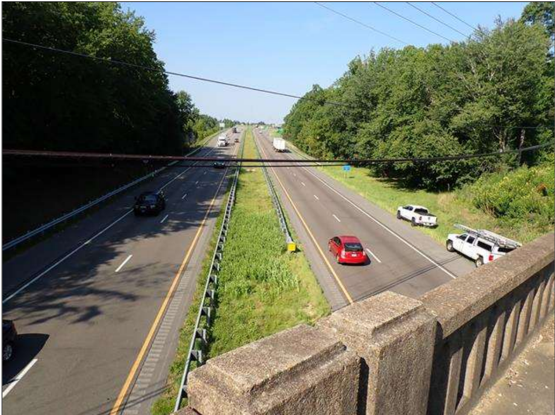
roadway looking west
