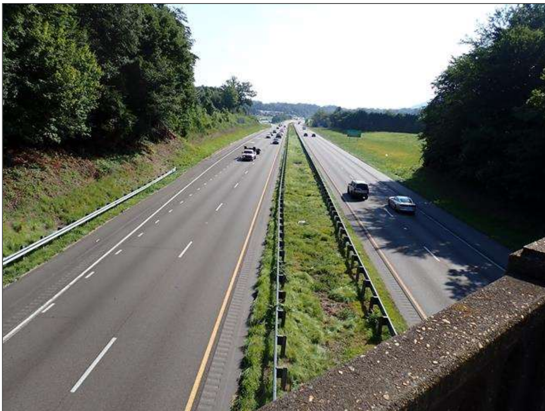
roadway looking east
