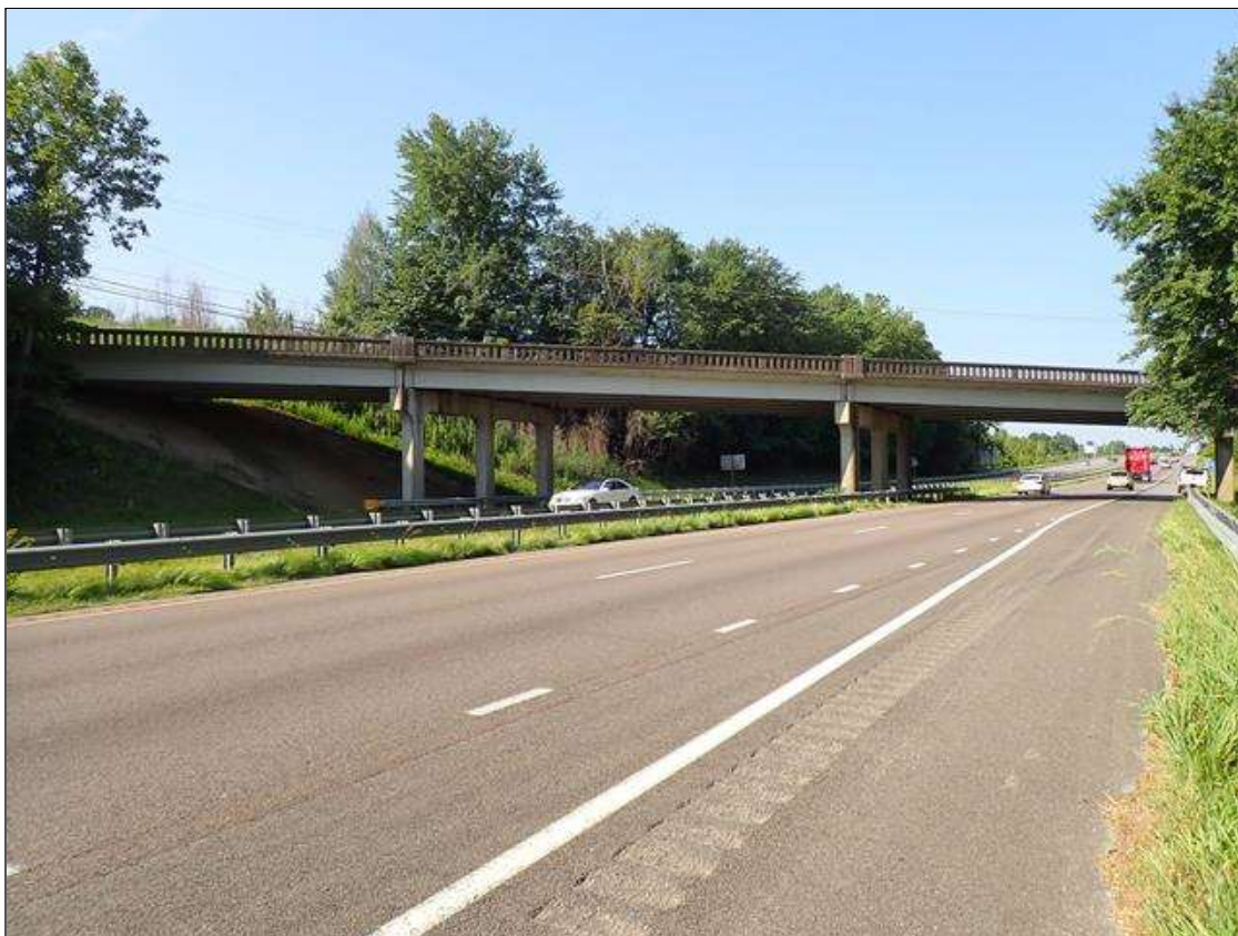
east profile looking west
