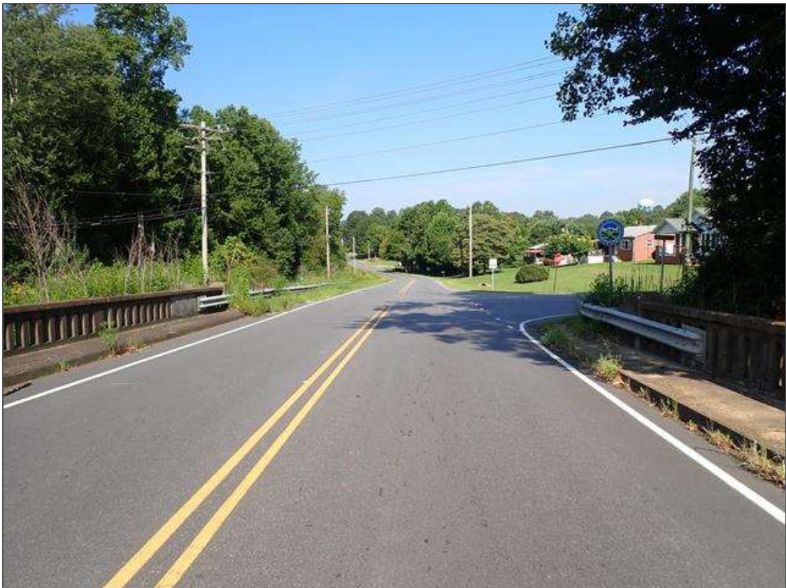
north approach looking north
