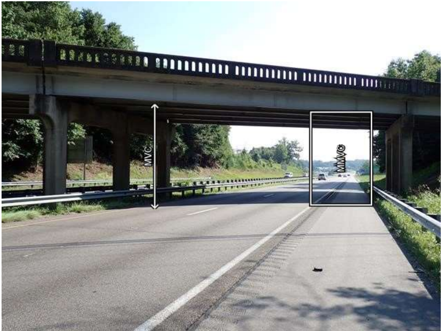
roadway under span 2, looking east
