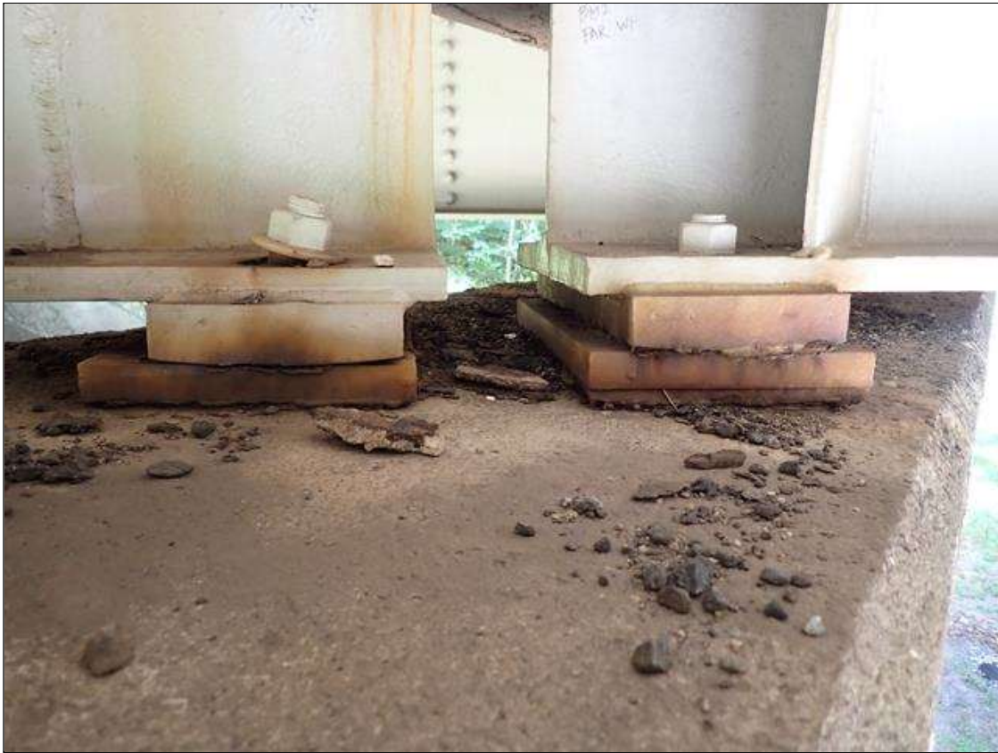
interior bearing assembly
