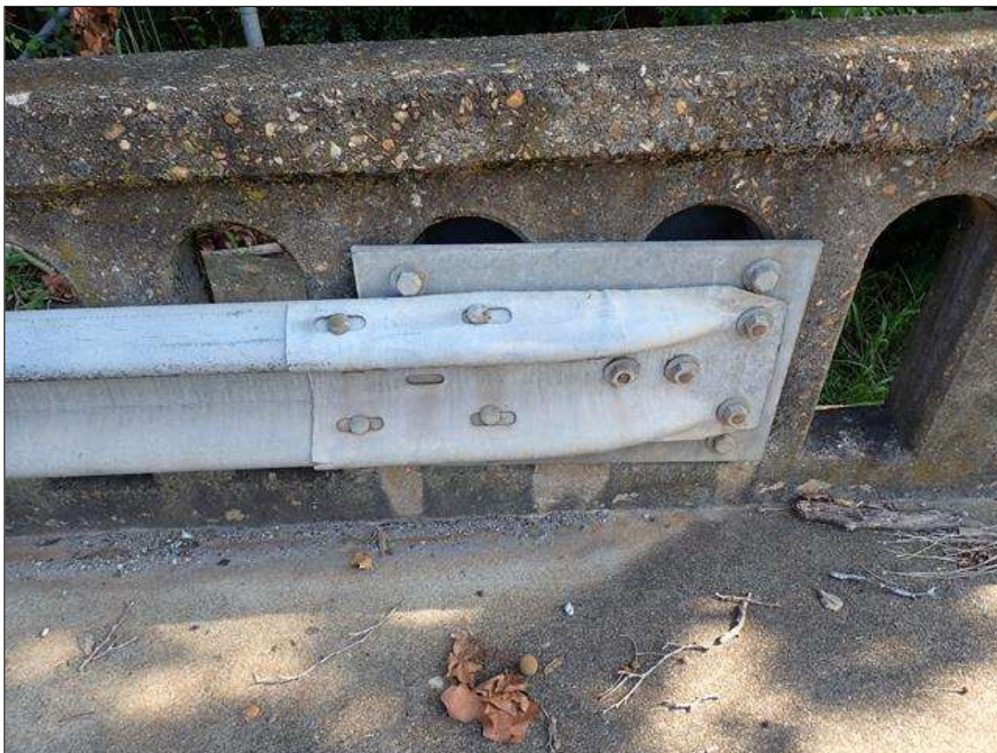
northeast guardrail attachment
