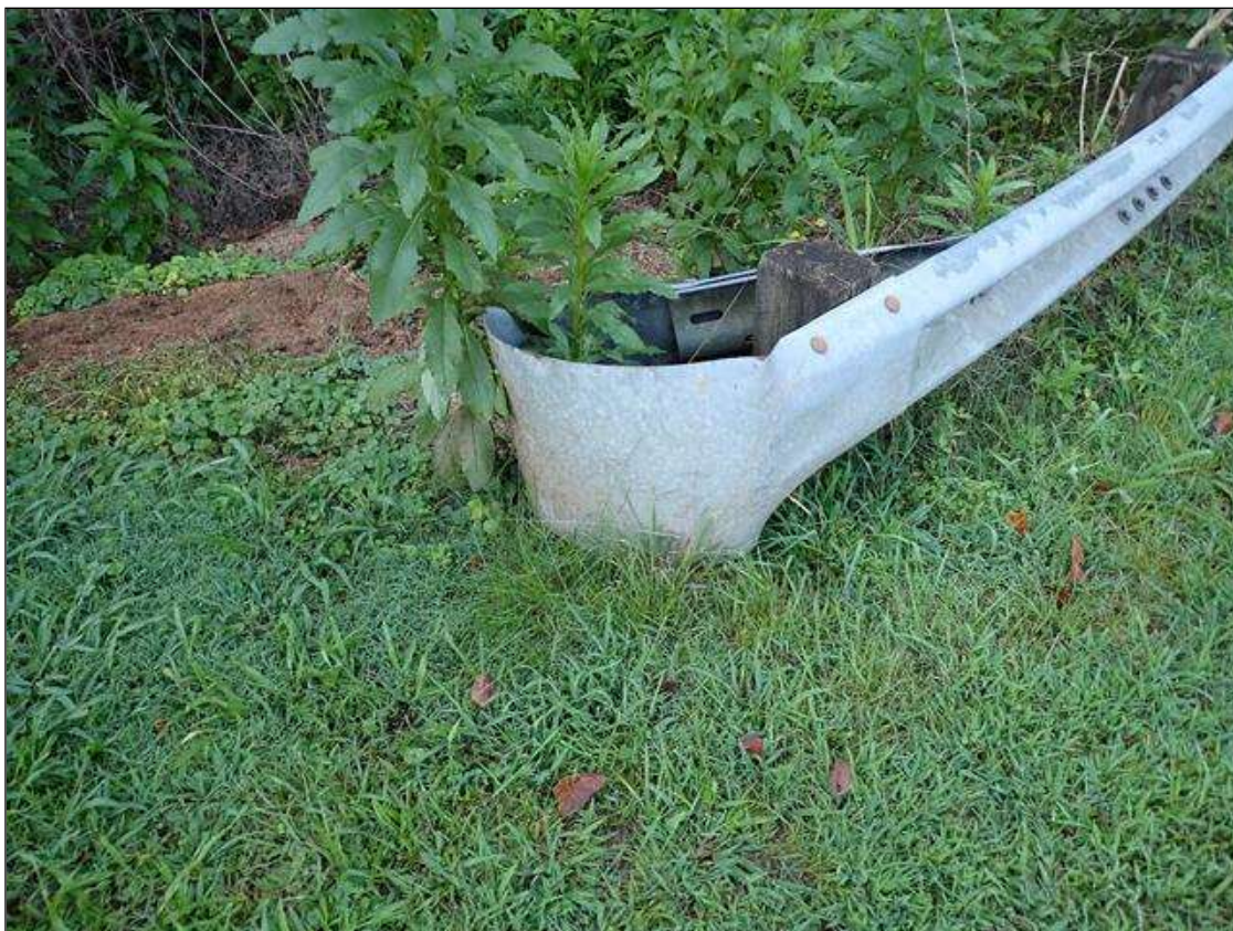
northeast guardrail termination
