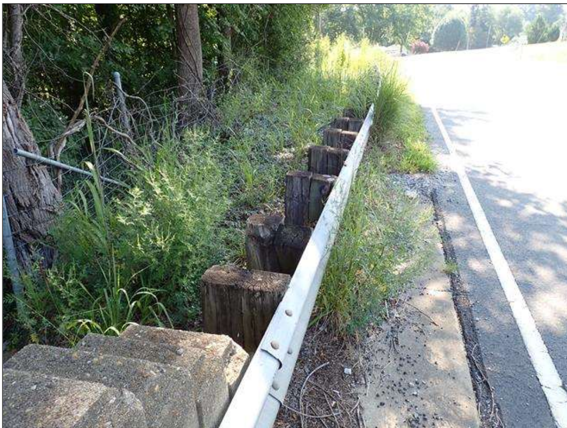
southeast guardrail transition
