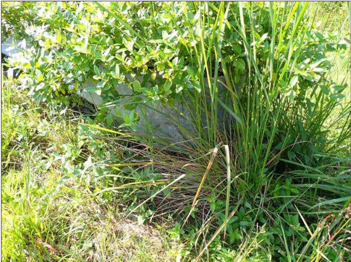
northwest guardrail termination
