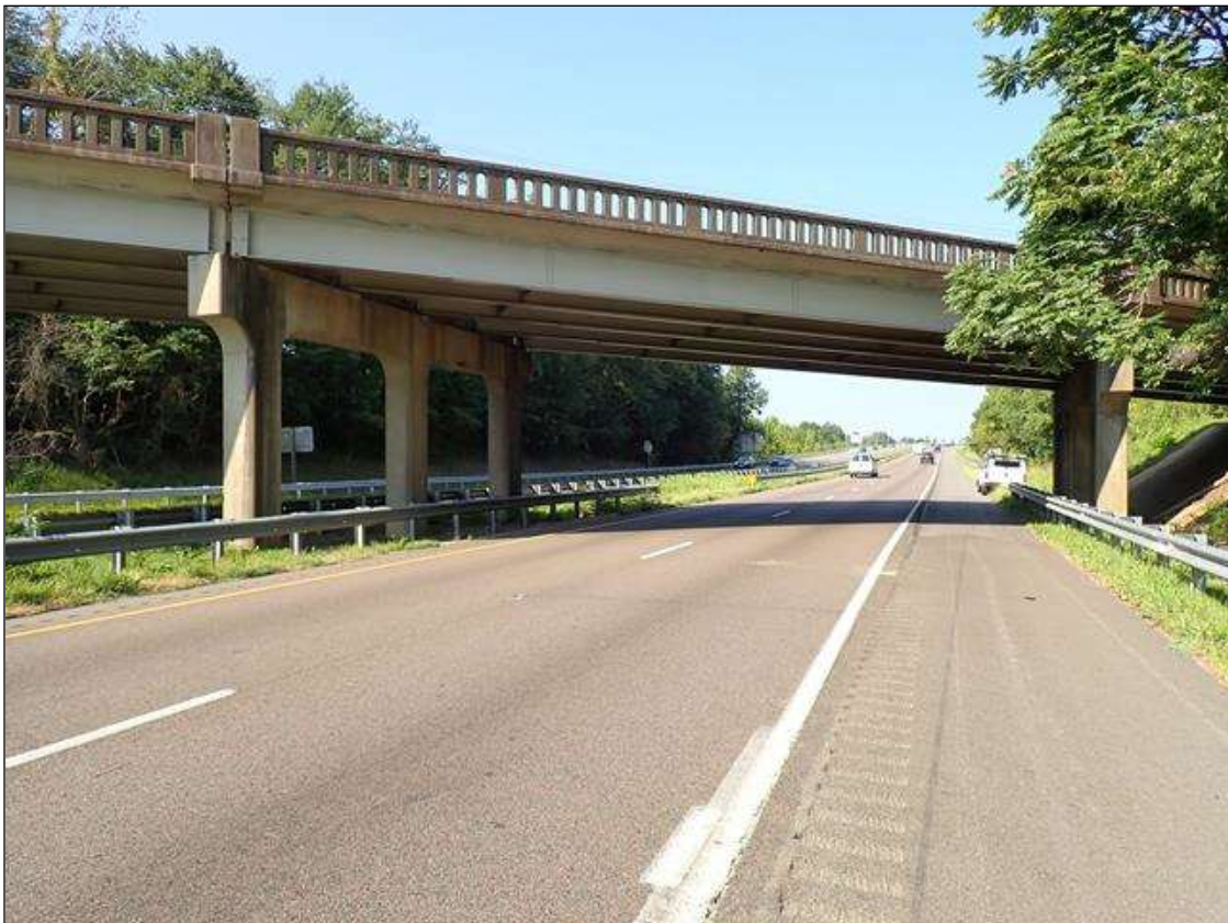
roadway under span 3, looking west (I-40 westbound)
