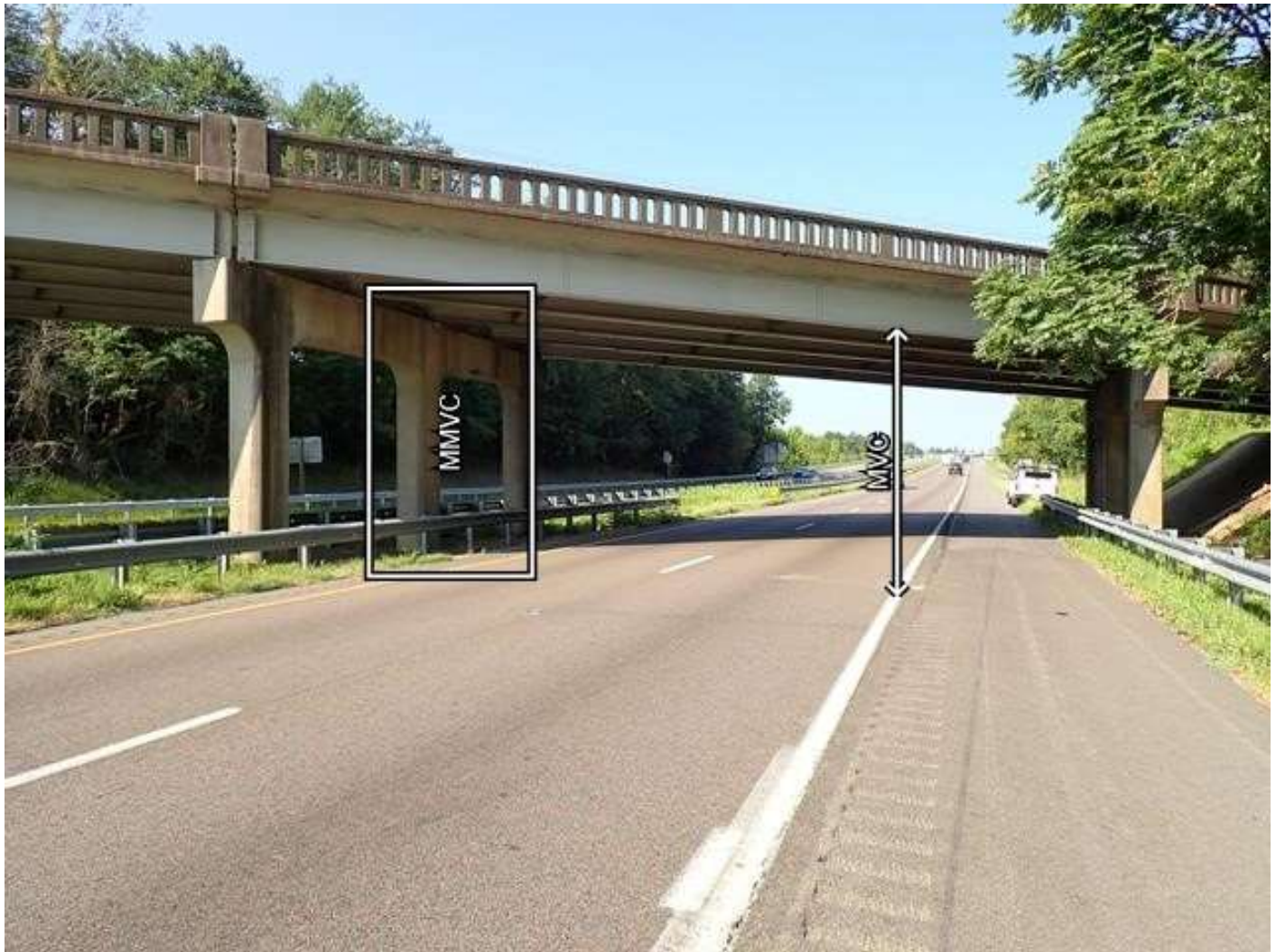
roadway under span 3, looking west
