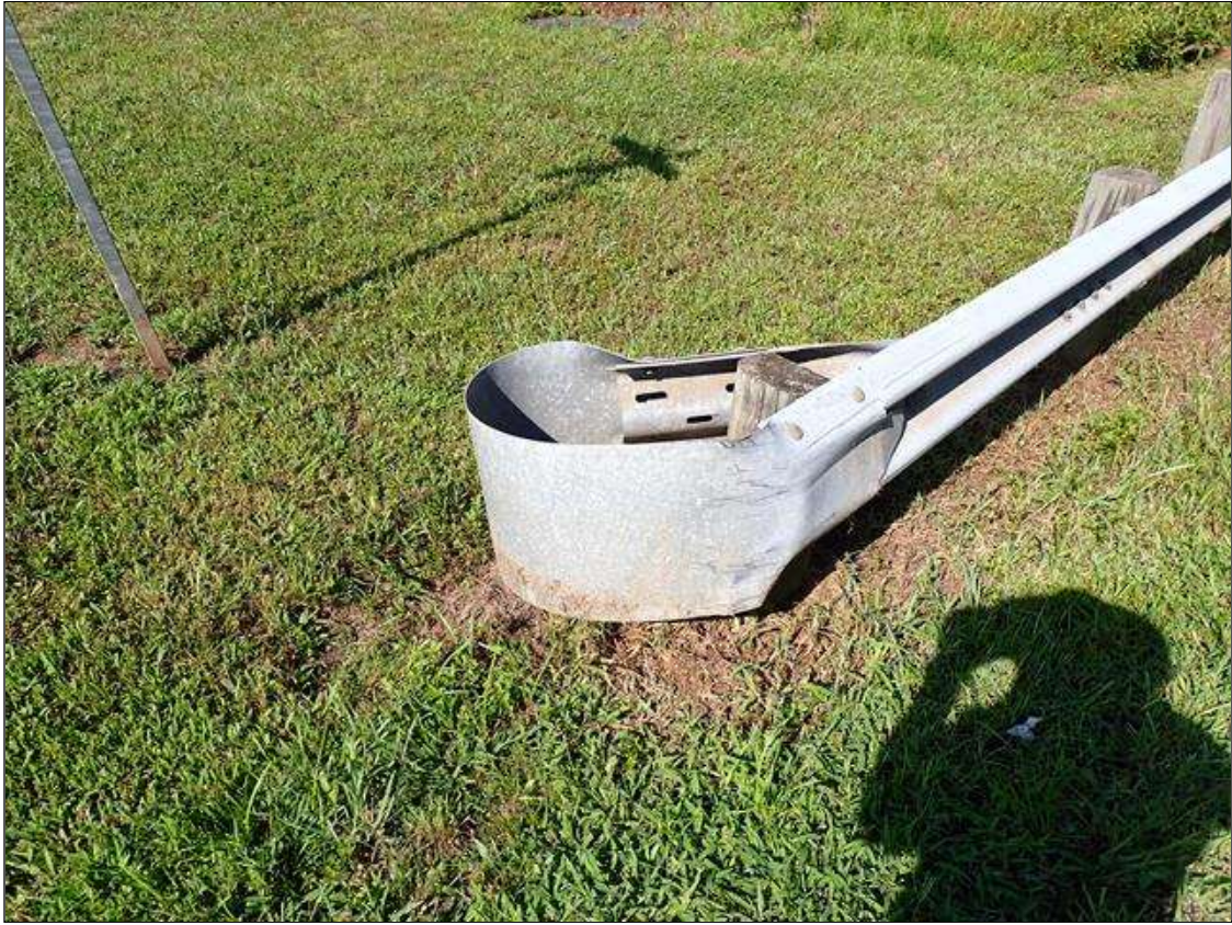
southwest guardrail termination
