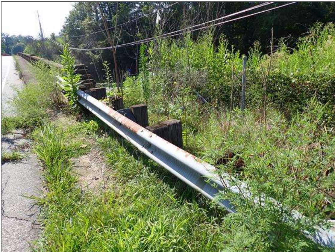
northwest guardrail transition
