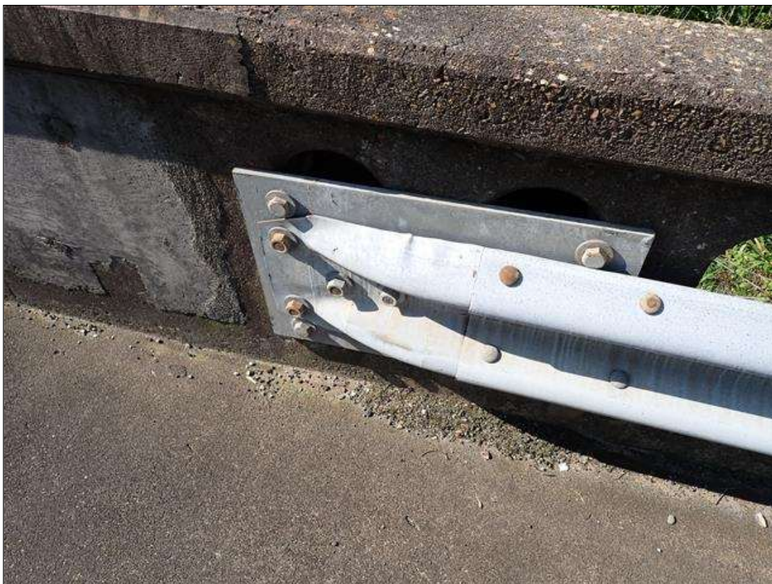
northwest guardrail attachment
